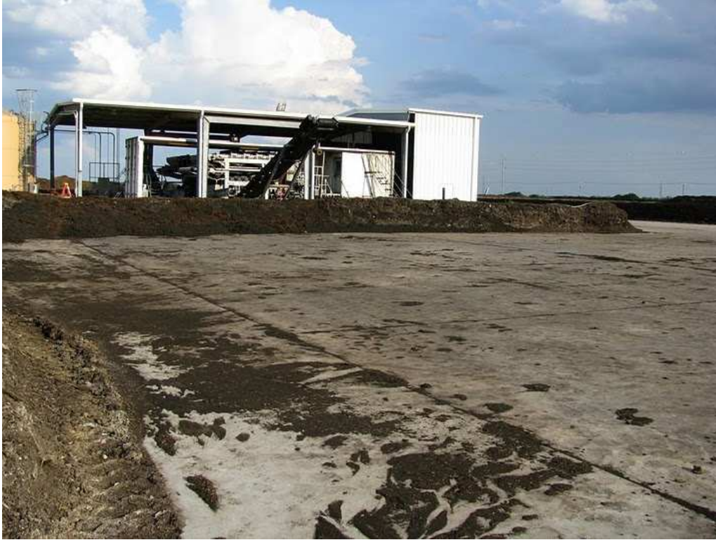
Photo of a concrete windrow composting pad, adjacent to a municipal wastewater sludge (biosolids) dewatering operation; These facilities are at a permitted municipal wastewater sludge treatment plant site.
